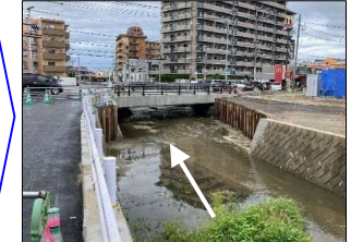
②周船寺橋架替橋長10.5m⇒20.5m
