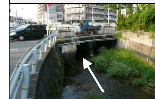
②周船寺橋架替橋長10.5m⇒20.5m
