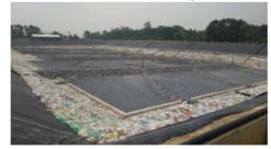
▲ Suppression of the generation of methane gas by aerobic bacteria due to ventilated structure of landfill
