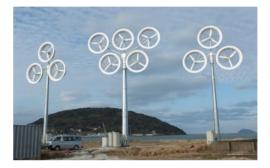
Example of the introduction of a multi-lens wind turbine
