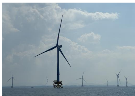
▲ Kitakyushu Hibikinada Offshore Wind Farm
