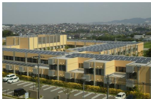
▲ Introduction of solar power generation at Fukuoka Prefecture Dazaifu schools for special needs education
