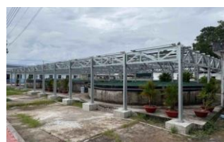
▲ On-site installation in Vietnam
